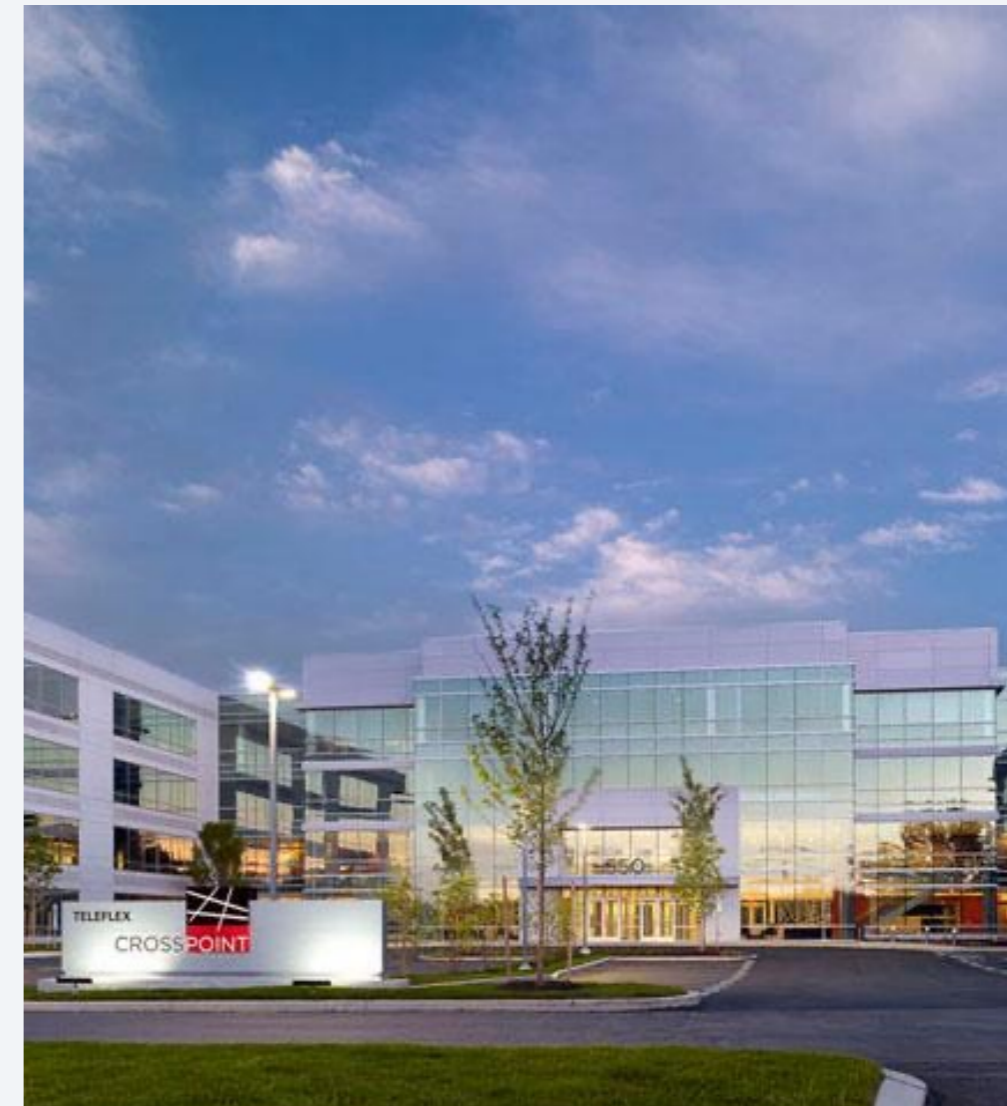
Our Global Headquarters office in Wayne, Pennsylvania is a UL Verified Health Building for Indoor Air, and it is LEED Gold and Energy Star certified.
